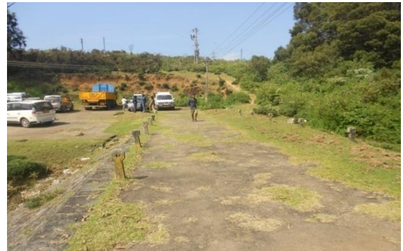
Earthen Dam top to be provided with screed concrete at top for drainage
