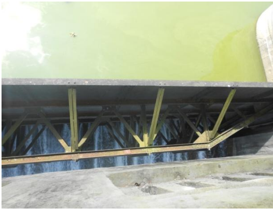
Spillway gate stiffener plates & Rubber seals to be replaced
