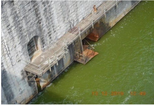
Scour vent outlet approach steel ladder and platform to be replaced including the sluice valve
