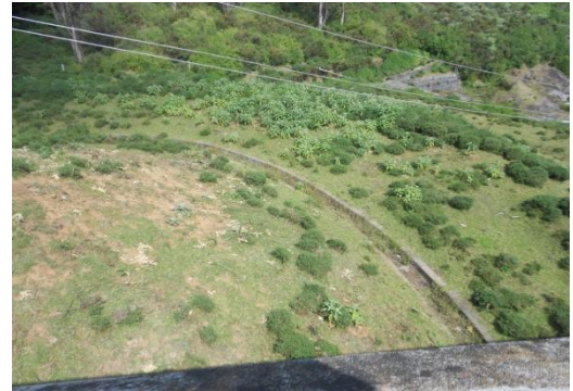
Downstream side chute drains to be provided in turfed portion
